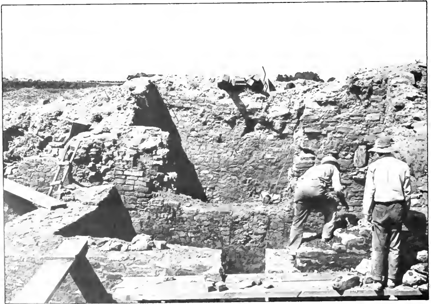
Figure 12.2. Two views of wall repairs, West Ruin, by American Museum of Natural History crews.
